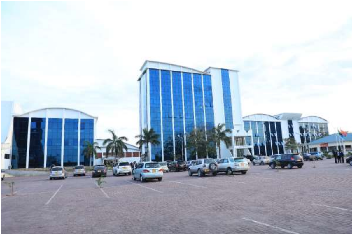
Picture 1: The LST Buildings Located in Plot No. 2005/2/1 Off Sam Nujoma Rd/Mpakani Rd
