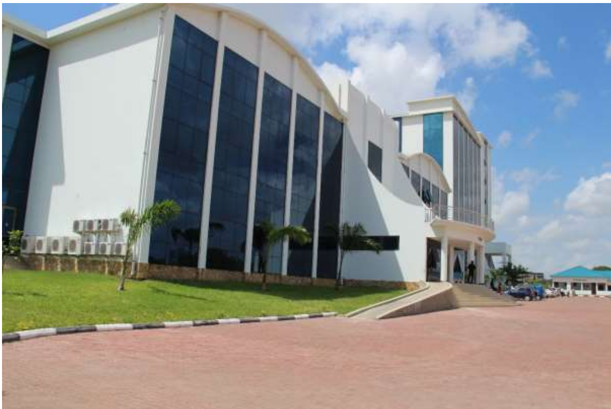
Picture 2: The LST Library Building
